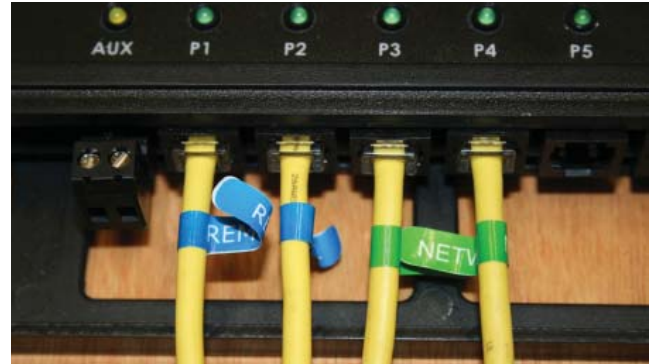
Figure 2-7, Surface Mounted Remote/Network Cables
