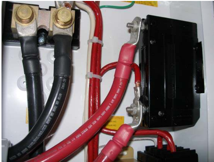
Battery Positive connections and shunt wiring
